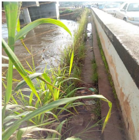
Plate 3.2 Walkway without rails to prevent from falling into the river.
