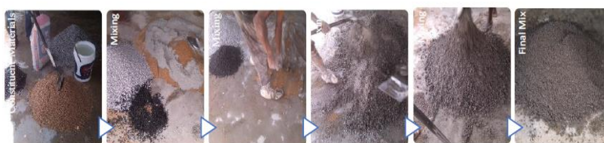
Figure 3: Mixing of Fresh Crumb-Rubber Masonry Concrete for Block Production
