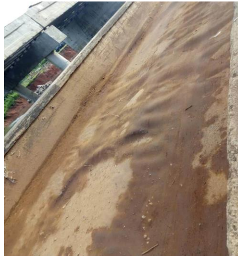
Plate 3.3 Top of the bridge deck with superimpose deteriorated layer
