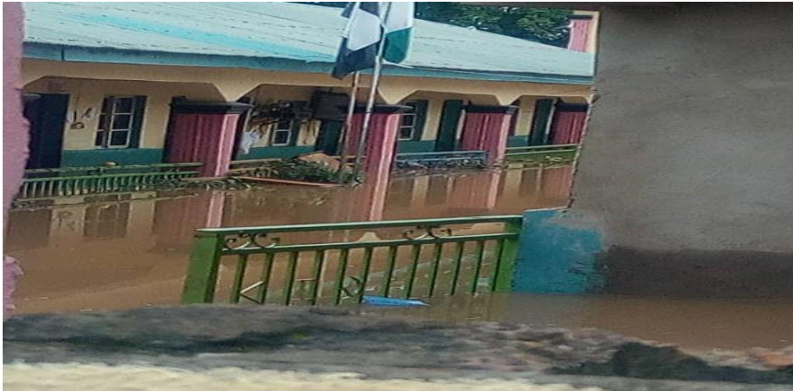
Plate 3: Adekids School flooded along the river Gbodofon flood plain in Osogbo.
