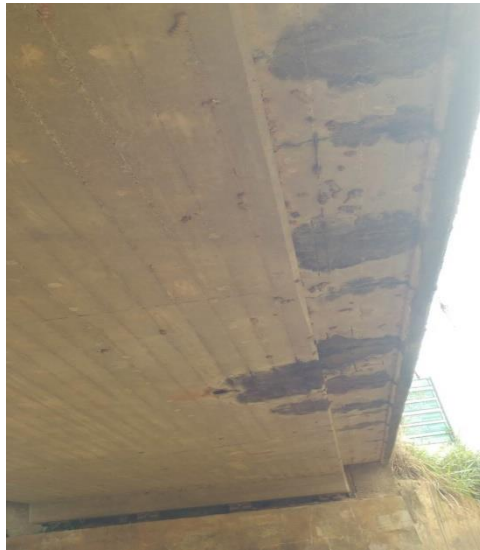
Plate 3.1 Distress under the bridge deck and corrode reinforcement as a result of concrete cover spilled off.
