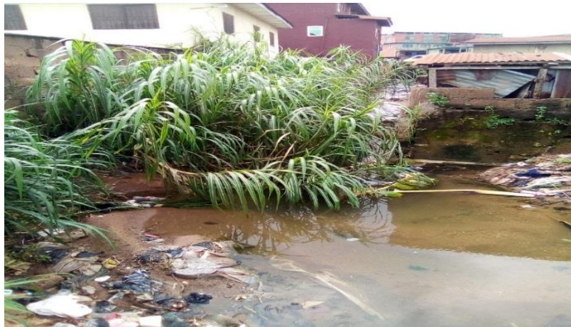
Plate 4: Dredged area blocked with waste behind Old-garage Motor Park.
